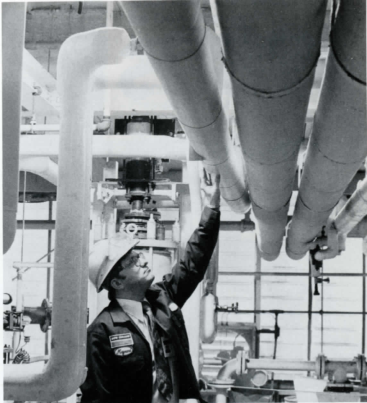
Energy conservation was a much-talked-about issue in the 1970s. Maynard Chaussee, then Instrument Section Supervisor in Design Engineering, located a Condensate Receiver System that required better insulation on lines and tanks to contain heat. His idea saved the Midland Plant $25,000 annually.
