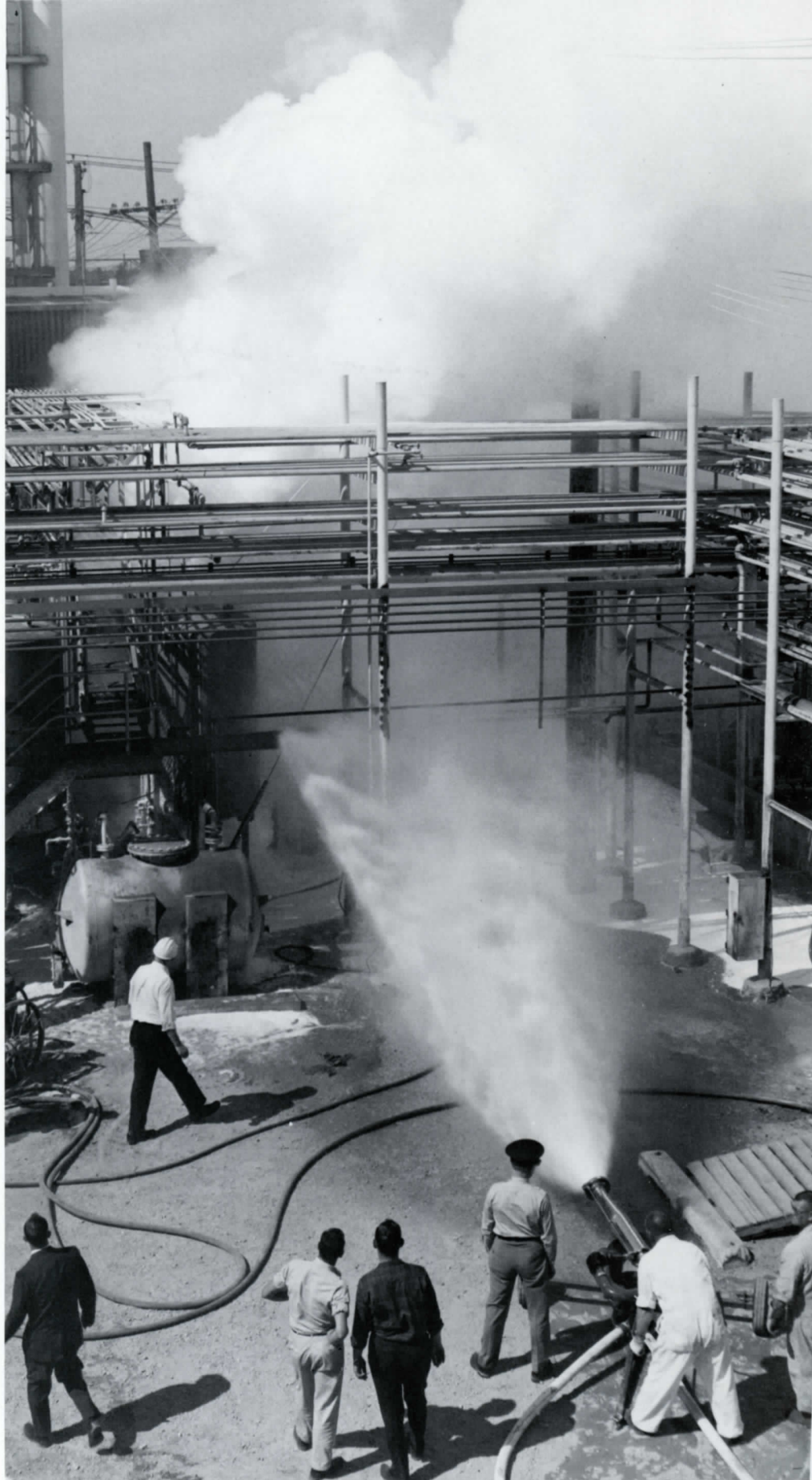
Dow Corning's safety performance is one of the best in the chemical industry. The Safety Department quickly foamed a spill in 1963 at 308 Building, caused by broken sight glass. Today, many reflex sight guages have been installed to alleviate the problem.
