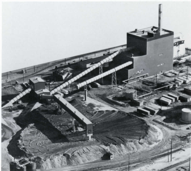
An overall view of the Midland Plant's Steam and Electric Cogeneration Power Plant that started up in December 1982. The 4½-acre woodchip pile is to the left of the SECO Plant. The tubes house the belt conveyors that bring wood to the power plant.
